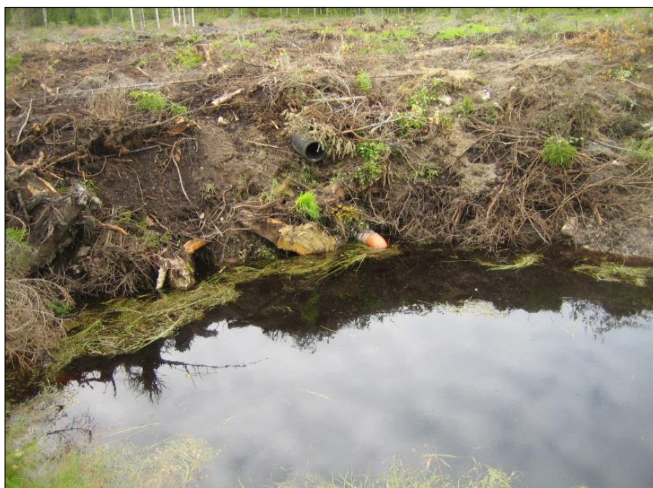
Figure 8. A peak runoff control structure in Finland. The lower pipe is orange and the upper pipe is black. Photo by Antti Leinonen.
