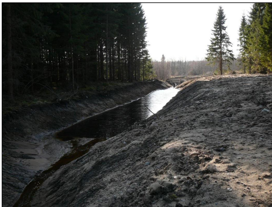
Figure 6. A sedimentation pond in Latvia. Photo by Zane Libiete.
