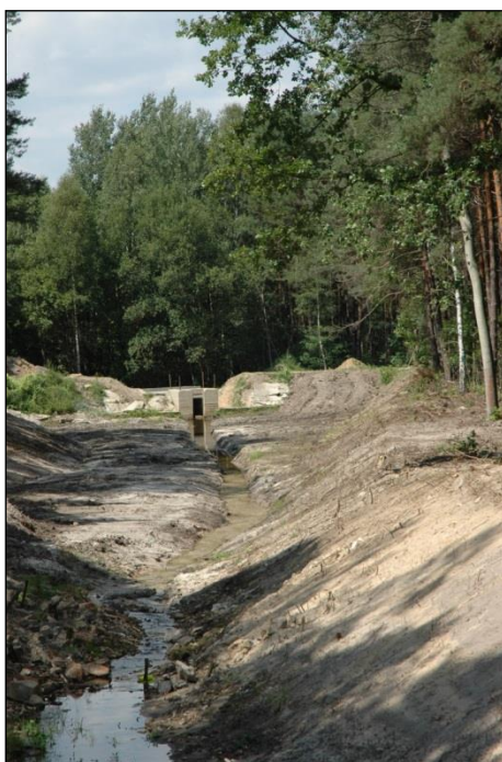
Figure 3. A water retention dam in a Polish ditch network. Photo by Wojciech Gil.
