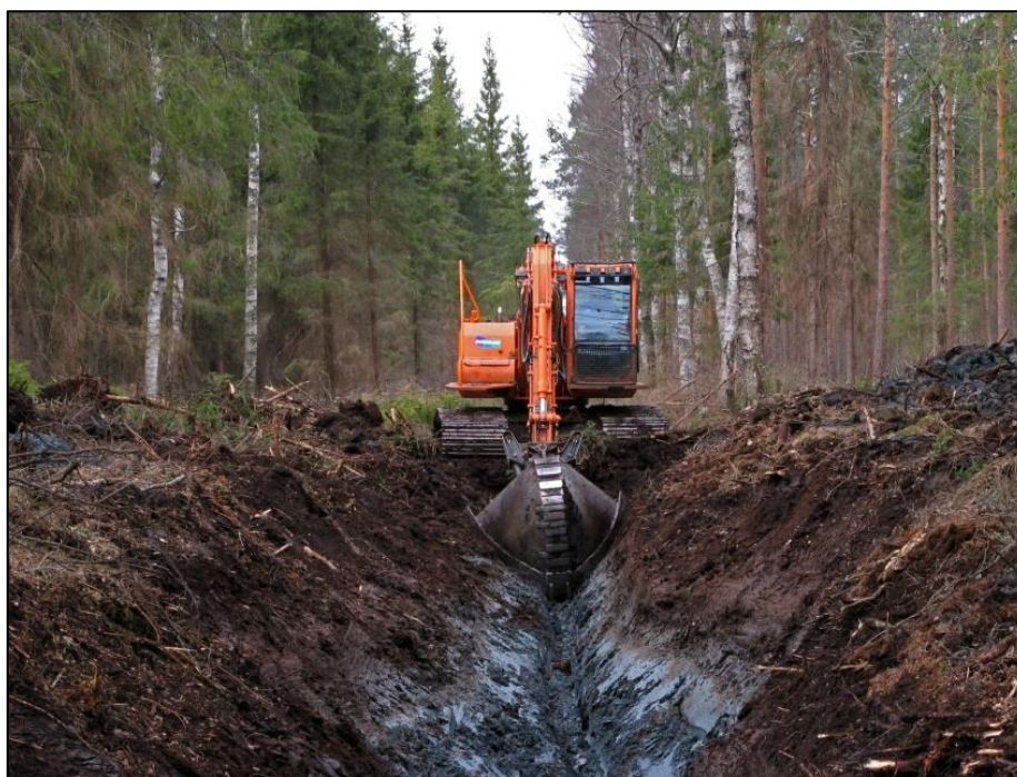
Figure 12. Ditch network maintenance in Finland. Photo by Markku Saarinen.
