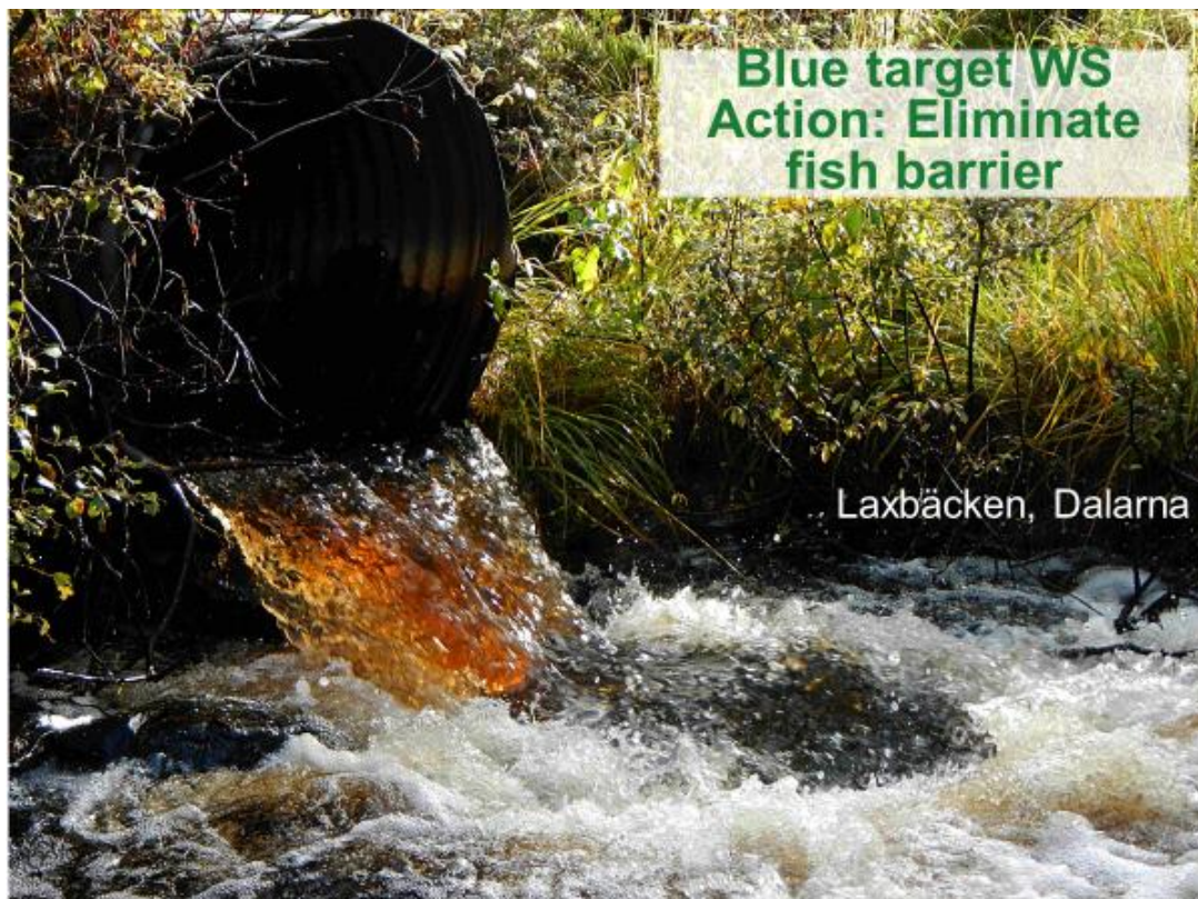
Fish and benthos migration barrier. Blue target WS - Water requiring Special action.
