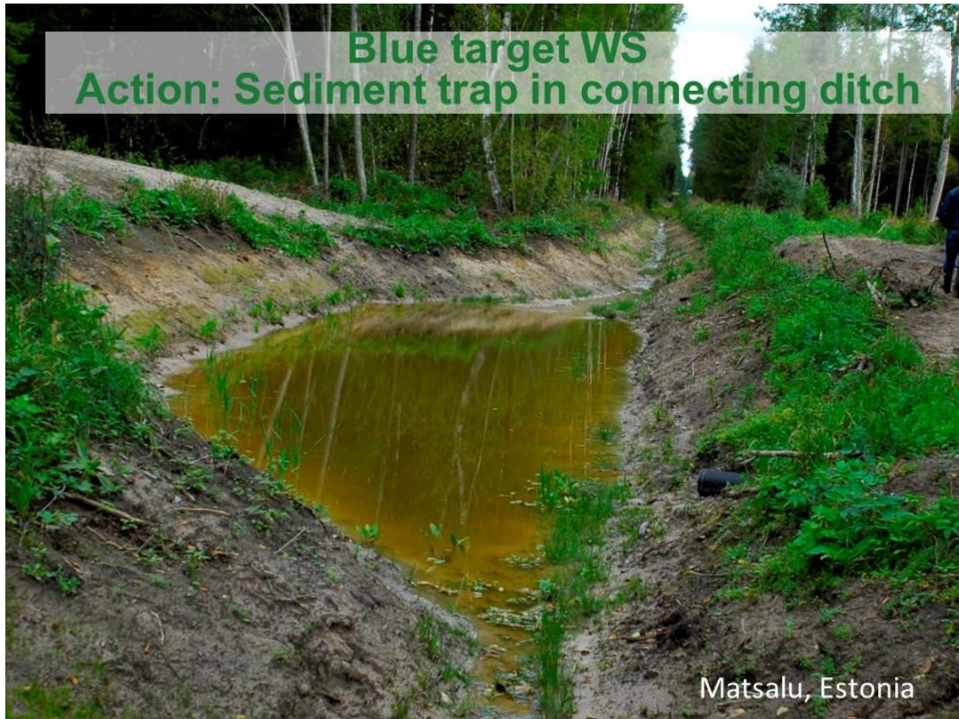
Most of the sediment input from a connecting man-made ditch to the main stream is captured in a sediment trap. The main stream section has the Blue target WS - Water requiring Special action.
