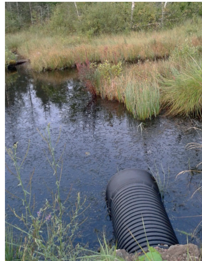
Figure 9.4. Installation of pipes against road flooding in beaver site in Lithuania. Photo: Olgirda Belova.
